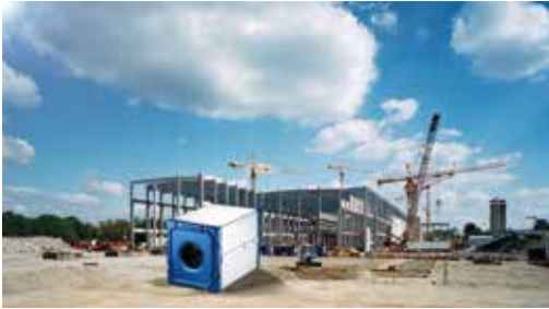
Construction machinery and cranes
