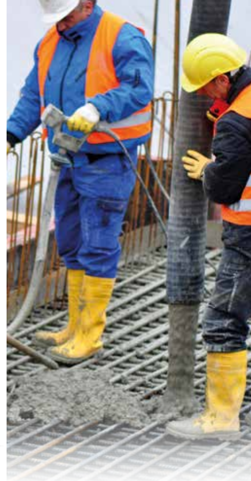
Fast and precise placement of the concrete pump.
