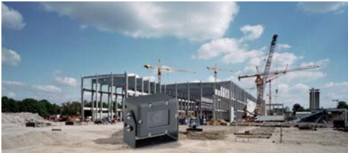
Construction machinery and cranes
